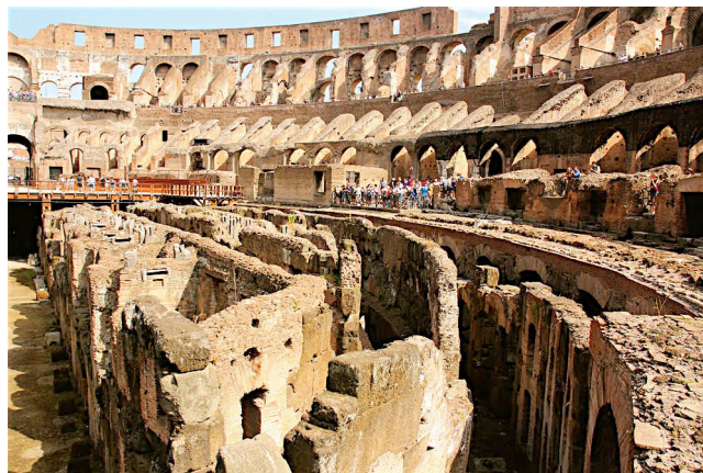
8.7 Construction of the Colosseum in Rome, Italy, was completed in AD80, but its stability is now threatened by accelerated weathering and erosion caused by acid rain.
